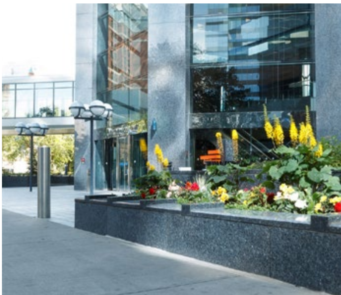
The façade of Devon Tower in Calgary is clad with Lundhs Royal Blue, which is a type of larvikite. Photo: Sean Phillips
