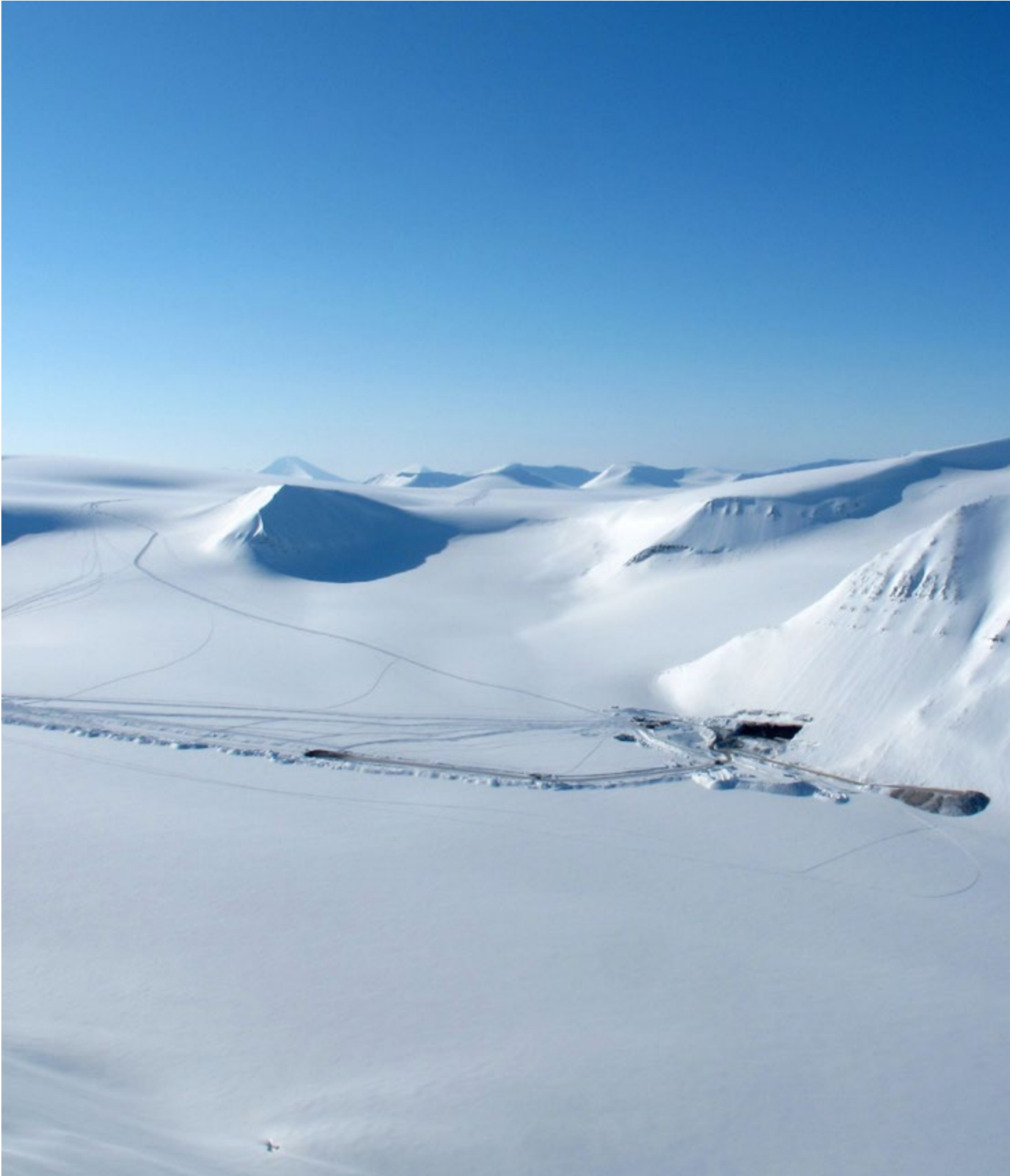
View from the Lunckefjell plateau towards the south across Martha Glacier where we see the exit from the Svea Nord mine at the base of Skollfjell and the road that has been begun across the glacier towards the opening on the Lunckefjell side of the glacier. Photo: SNSK, Malte Jochmann
