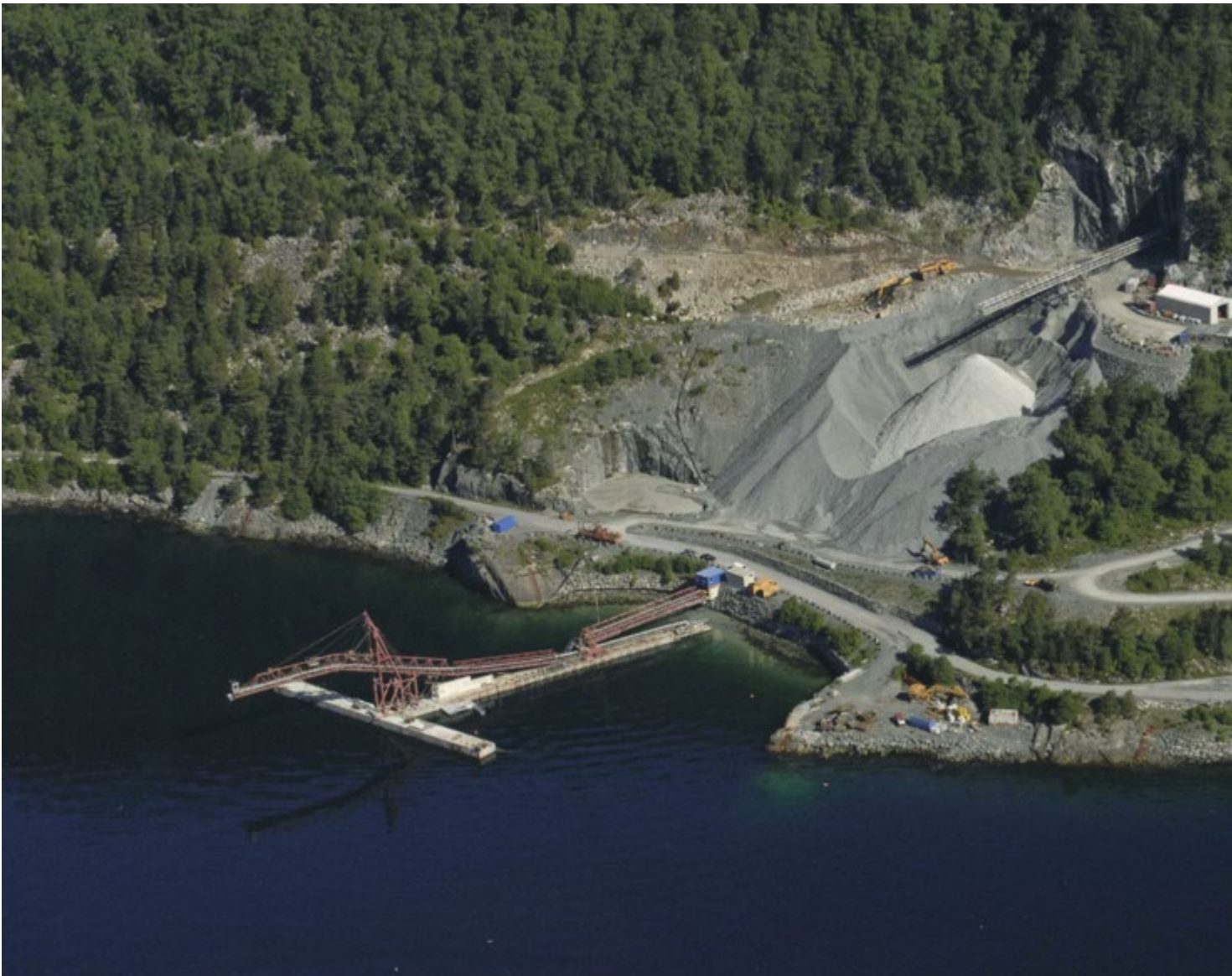
In 2011, Bremanger Quarry in Sogn og Fjordane exported 3.3 million tonnes of crushed stone to, i.a. the Netherlands and Belgium. The company has a CO 2 -friendly crushing method that involves releasing the stone from 200 m height in the mountains. The photo shows the plant at Dyrstad near Svelgen. Photo: Bremanger Quarry
