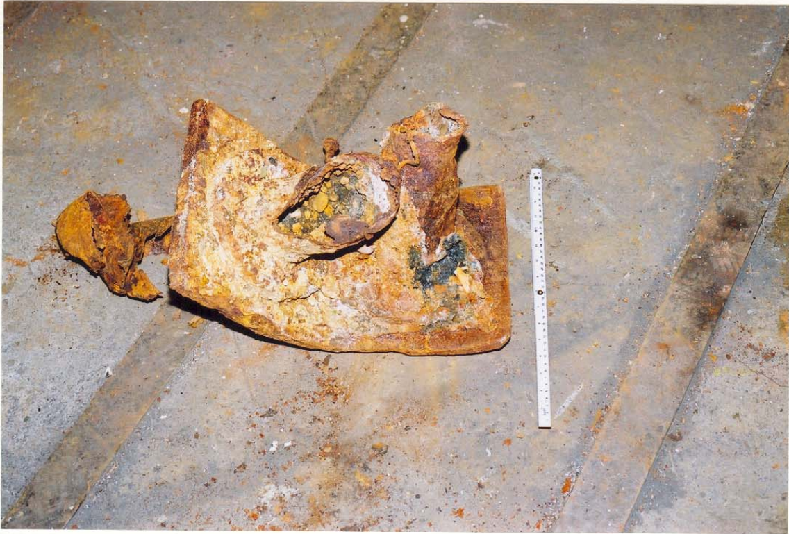
Figure 50 (1/24A): Deck doubler plate and trawl winch service pipes.
