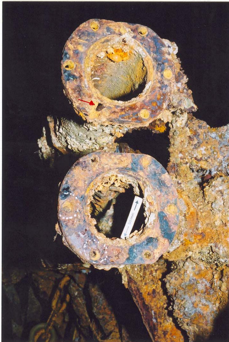
Figure 13 (8/13A): Exhaust flange connections showing retained studs (2 outlined in lower flange and one arrowed in upper flange).
