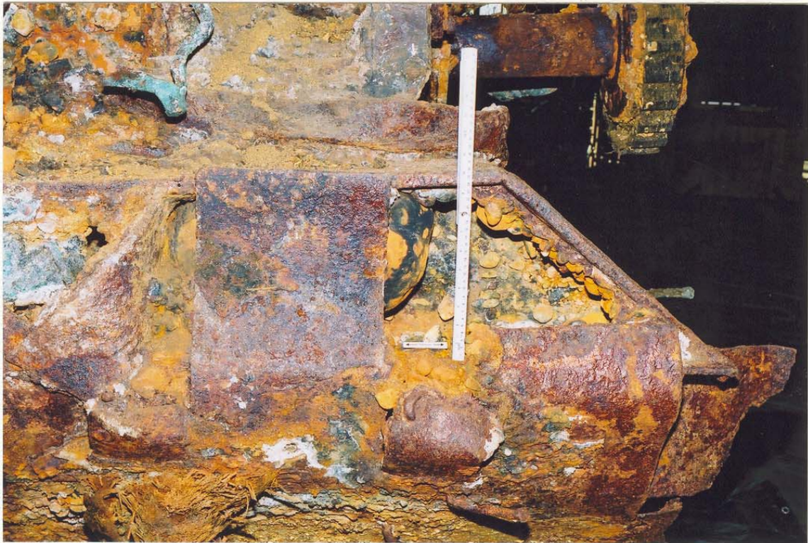
Figure 30 (03/7A): Detail of trapped pebble and backwardly deformed stiffener plate.
