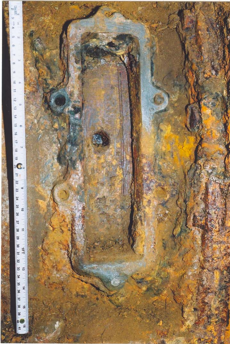
Figure 19 (8/10A): Detail of cam shaft drive cover location.
