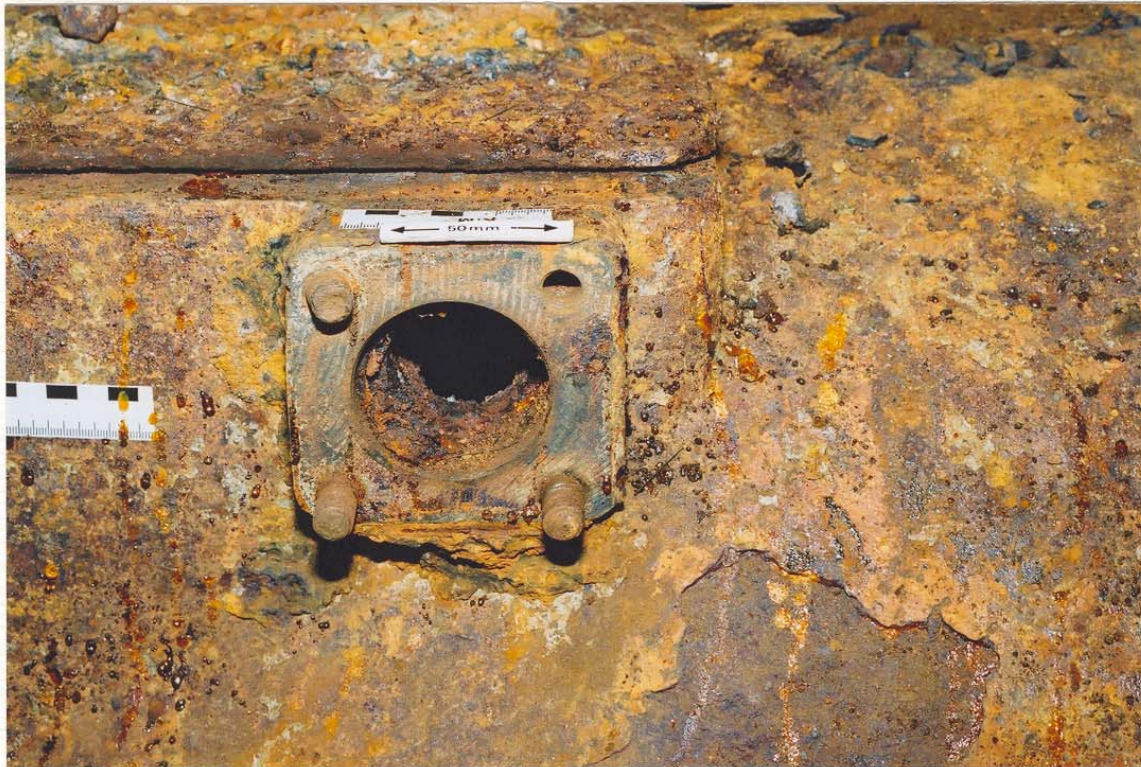
Figure 20 (8/11A): Detail of mounting flange shown in figure 18.
