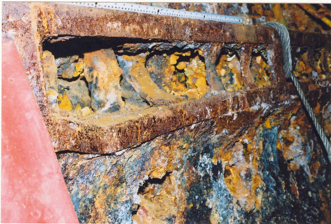
Figure 10 (8/1A): Detail of damage to charge air distributor.
