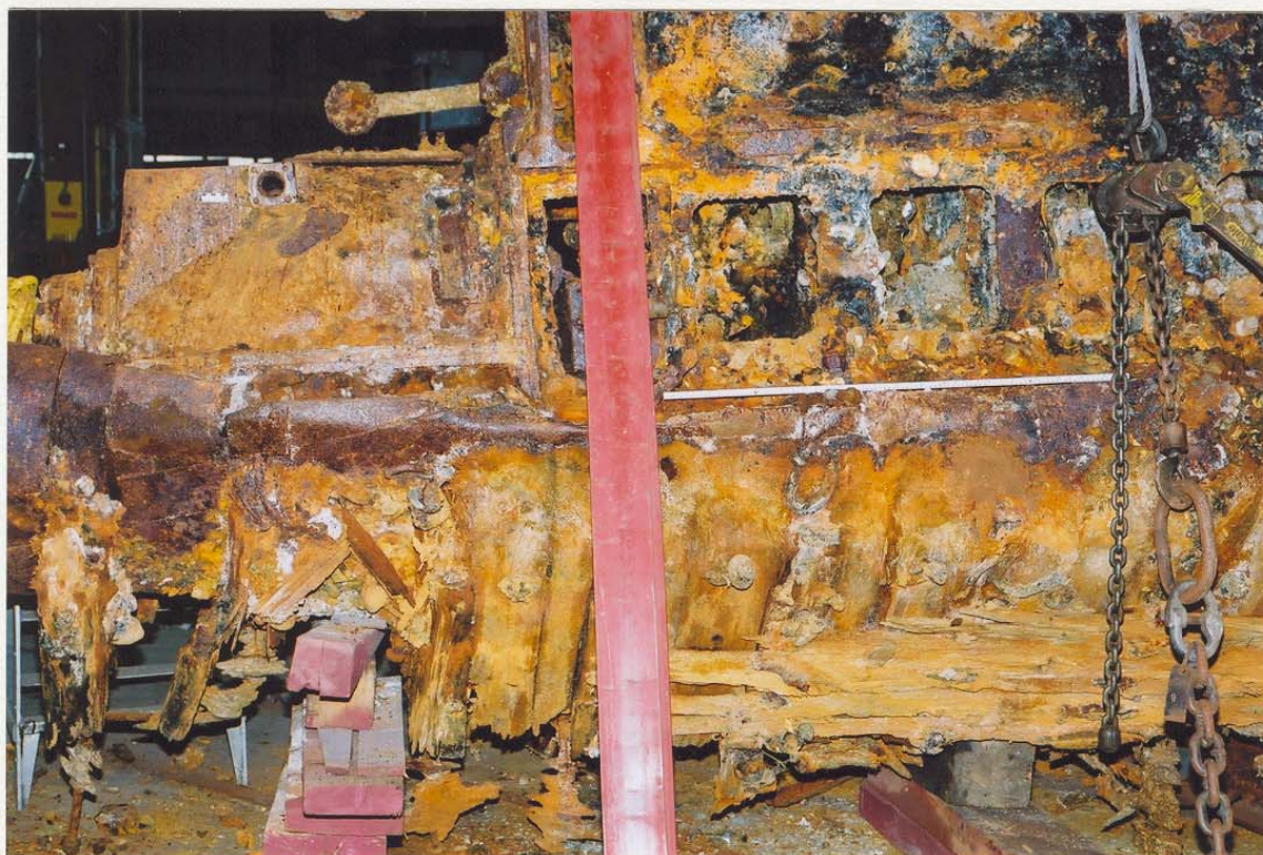
Figure 33 (03/13A): Engine starboard side showing upwardly bent foundation plates.
