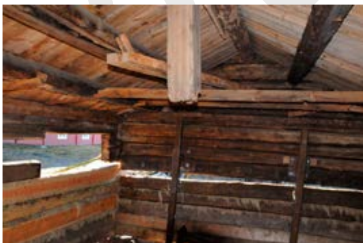
Stallen. Under restaurering (2010).
