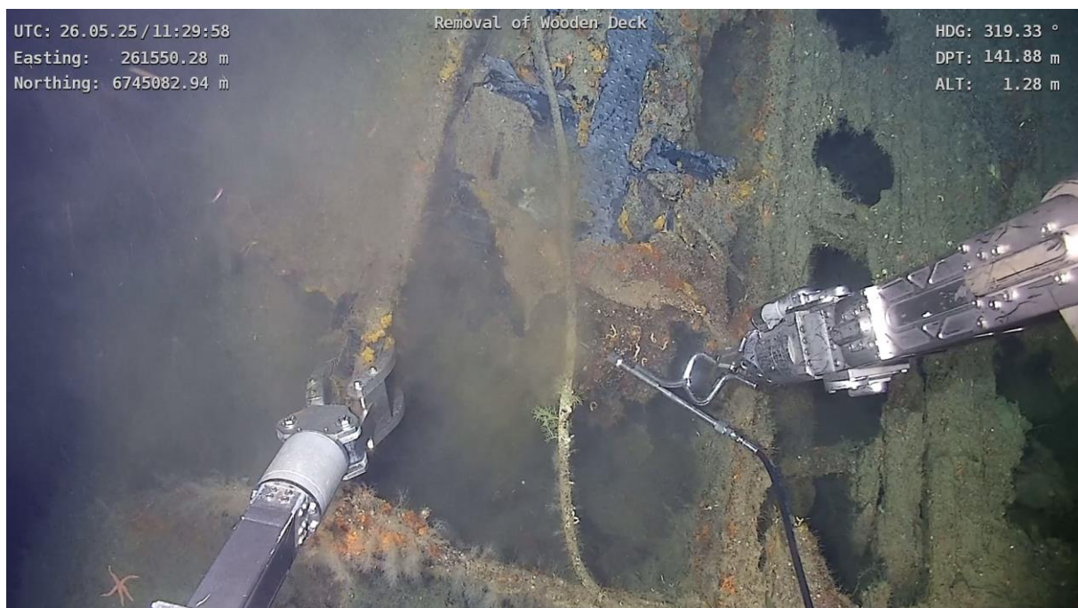
Figure 4-82 Water jet being used to clean debris from the opening at location 1
