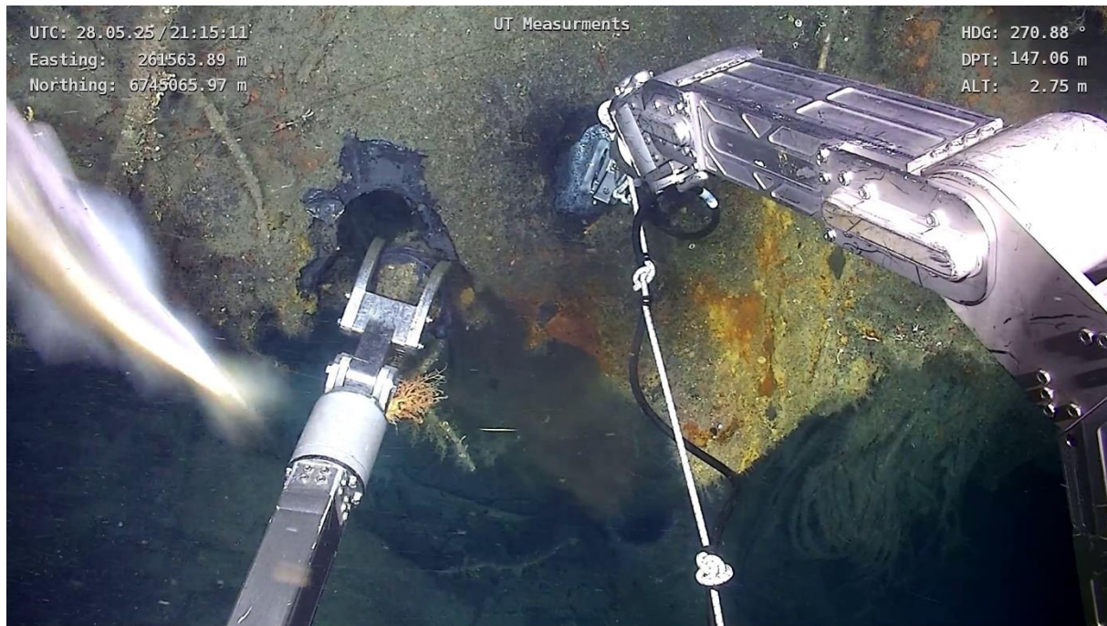
Figure 4-122 Ultrasonic measurement at location C
