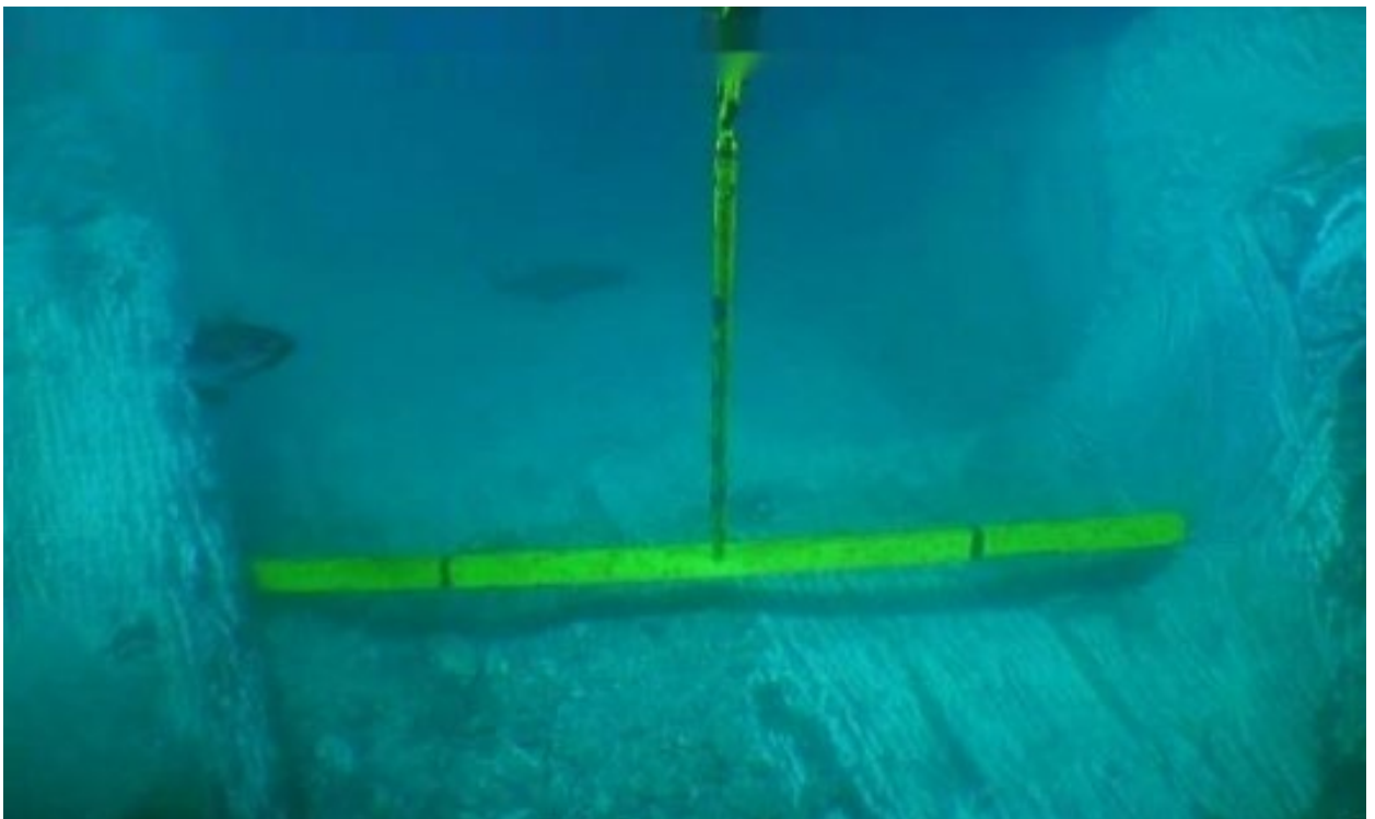
Figure 9-7: Subsea diggers can be equipped with dredging equipment, shear cutters and digging teeth's that can loose up and remove hard seabed and rock.
