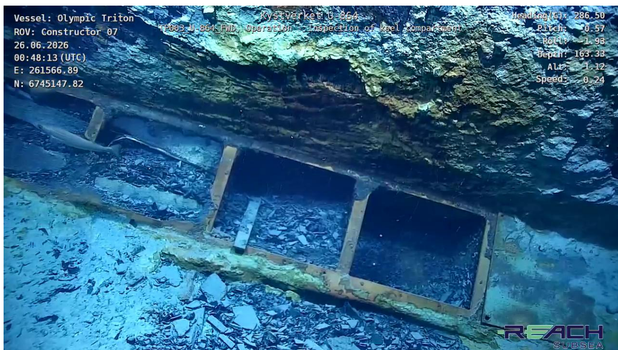
Figure 3-39 General visual inspection of the accessible compartments. Keel frame #60 to the right
