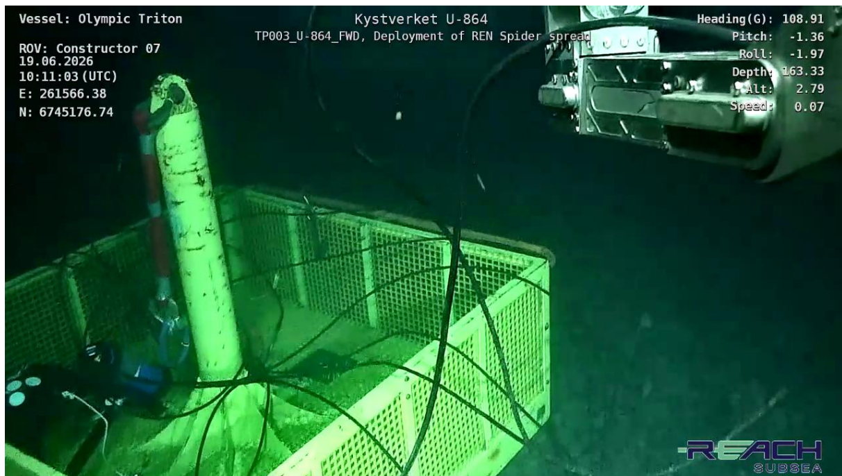
Figure 3-8 ROV hooking up three 80 m subsea cables for the ADCP and wreck monitoring Octans Inclination Sensors
