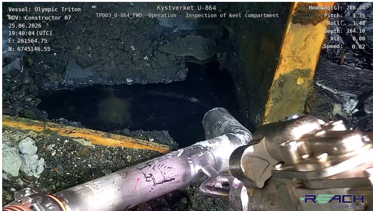
Figure 3-26 Recovery of liquid mercury from keel compartment
