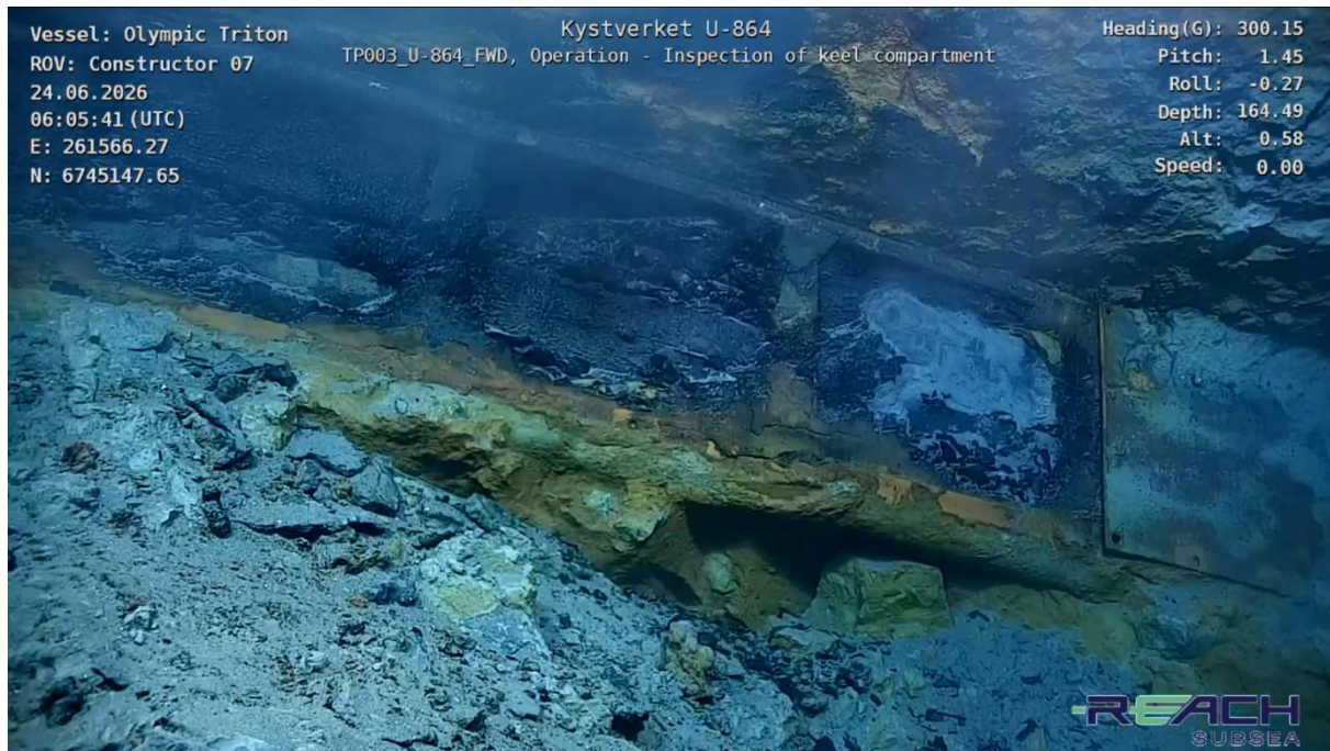
Figure 3-20 Keel compartments after removal of keel plate
