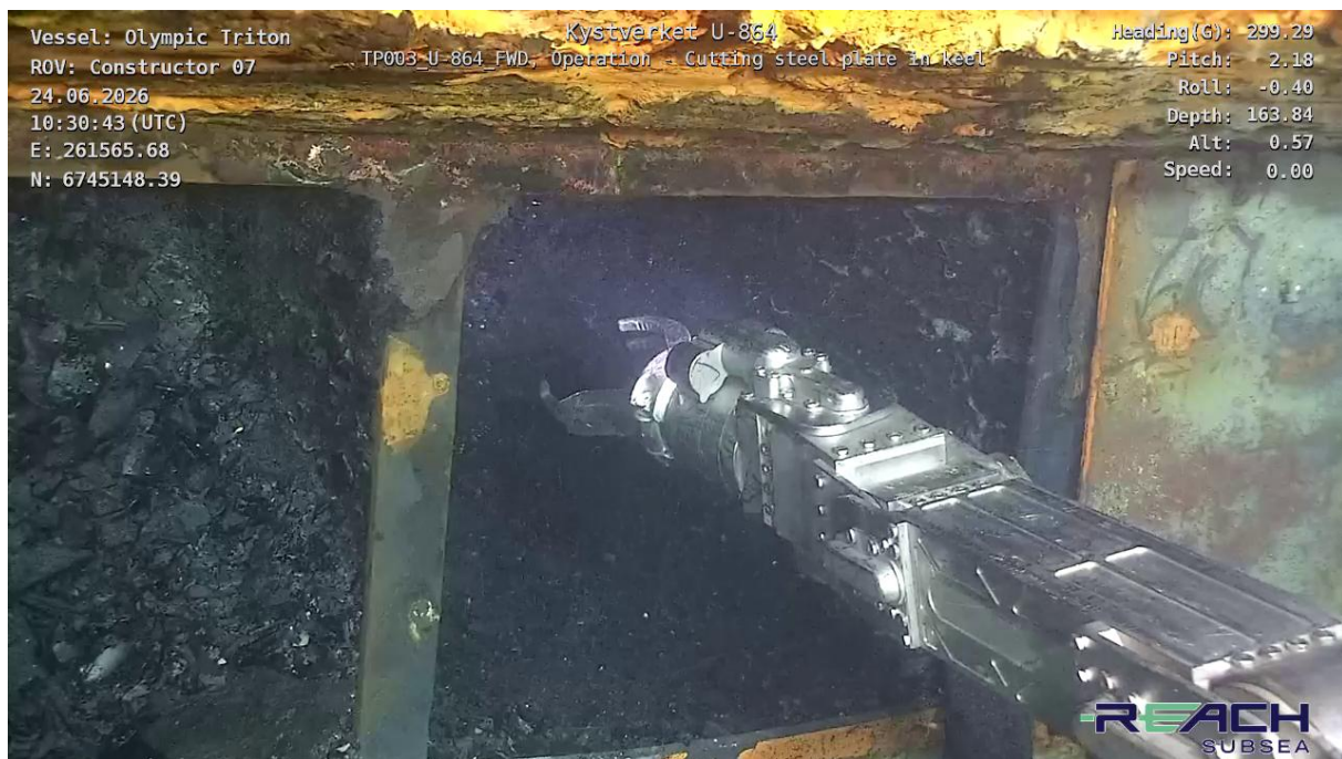
Figure 3-41 Inspection of first keel compartment #60-#61 (#103-#104) area
