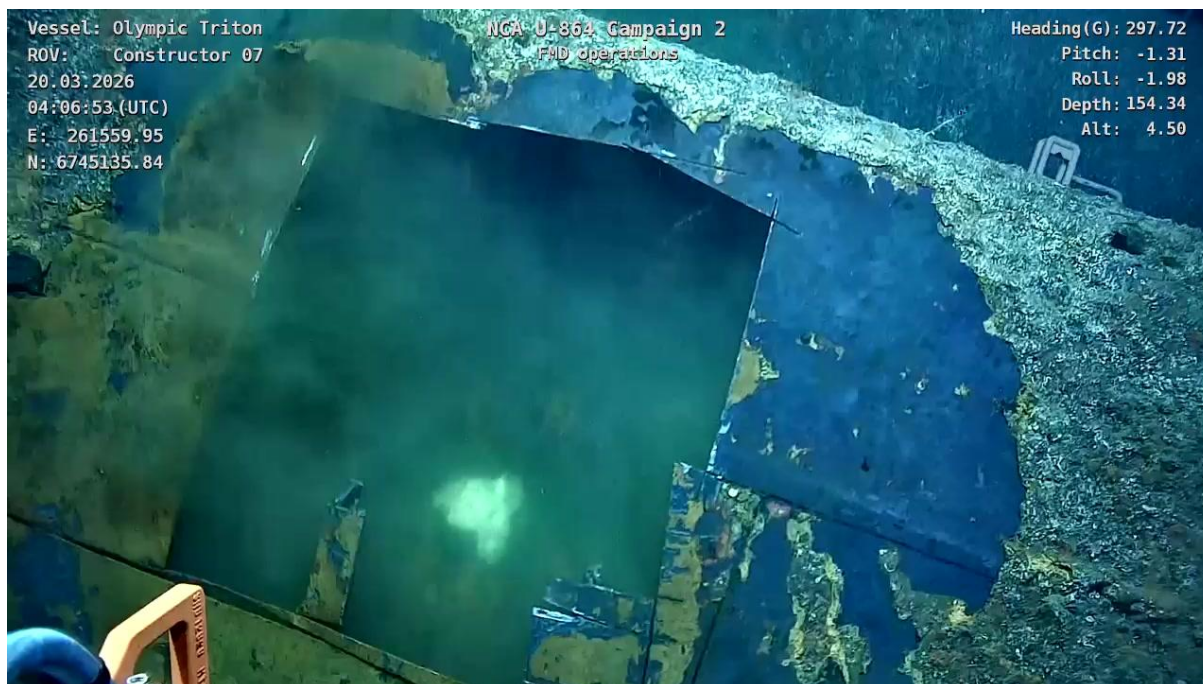
Figure 3-36 Post-cutting access of outer hull between frames #136-#138, allowing for FMD works
