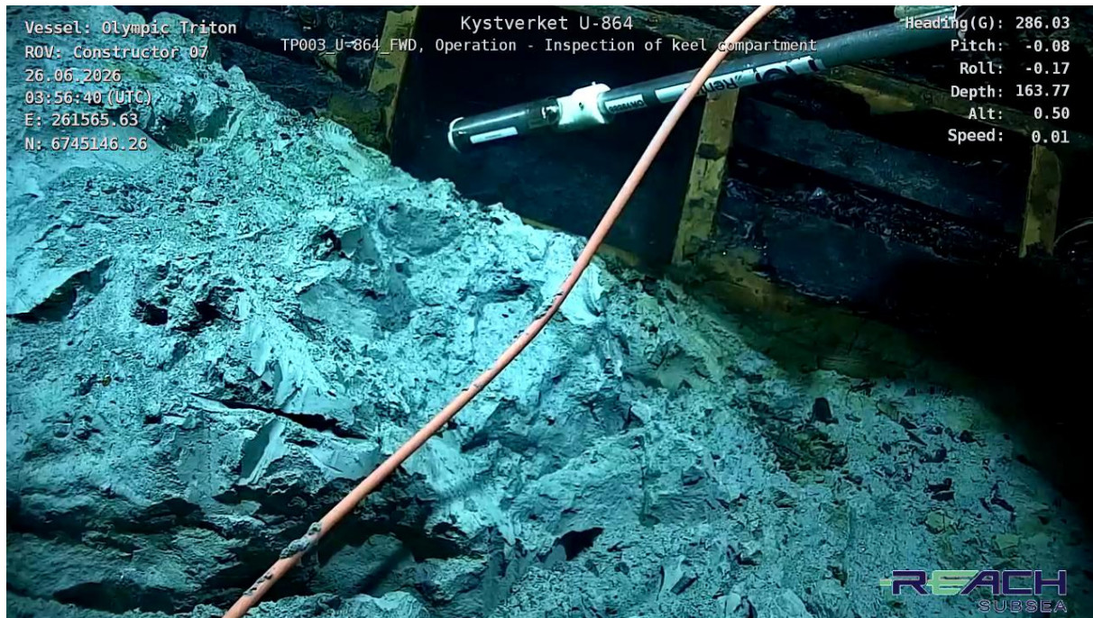
Figure 3-44 Camera stick used to inspect inside the keel compartment
