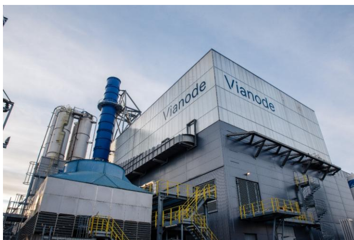
Figure 36 - Vianode's Via ONE plant at Herøya Industrial Park. (Photo: Vianode)
