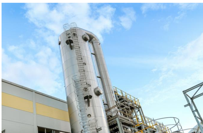
Figure 34 - REEtec's rare earth processing plant at Herøya Industrial Park. (Photo: REEtec)
