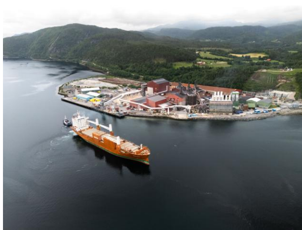
Figure 30 - Wacker Chemicals Norway's silicon metal plant at Holla. (Photo: Wacker)
