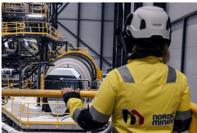
Figure 18 - Processing plant including crushing, grinding and separation of rutile and garnet concentrates. (Photo: Jostein Vedvik)
