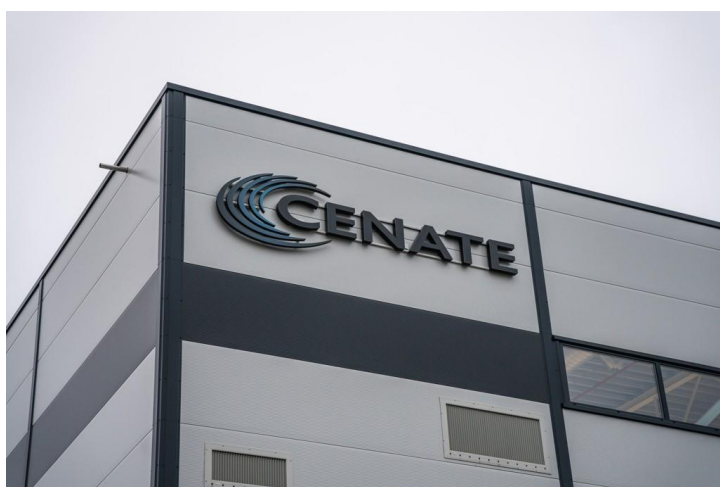
Figure 38 - Cenate's production facilities for silicon-based nanocomposite materials at Holtskogen in Tomter. (Photo: Cenate)
