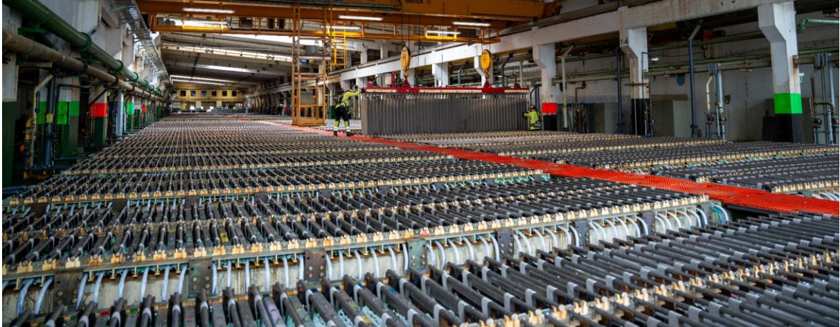
Figure 25 - The electrolysis hall where High Grade (HG) nickel metal is produced (Photo: Glencore Nikkelverk)
