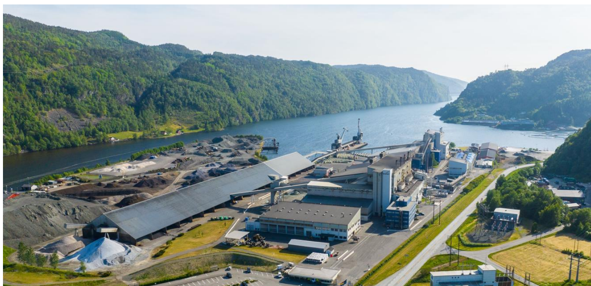
Figure 40 - Eramet's plant in Kvinesdal, where silicomanganese is produced. (Photo: Eramet)
