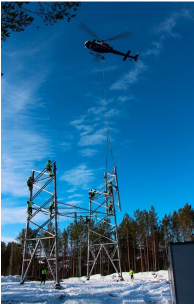
EFFICIENT POWER SUPPLY Construction of a new power line between Balsfjord in Troms County and Skaidi in Finnmark County PHOTO: STATNETT
