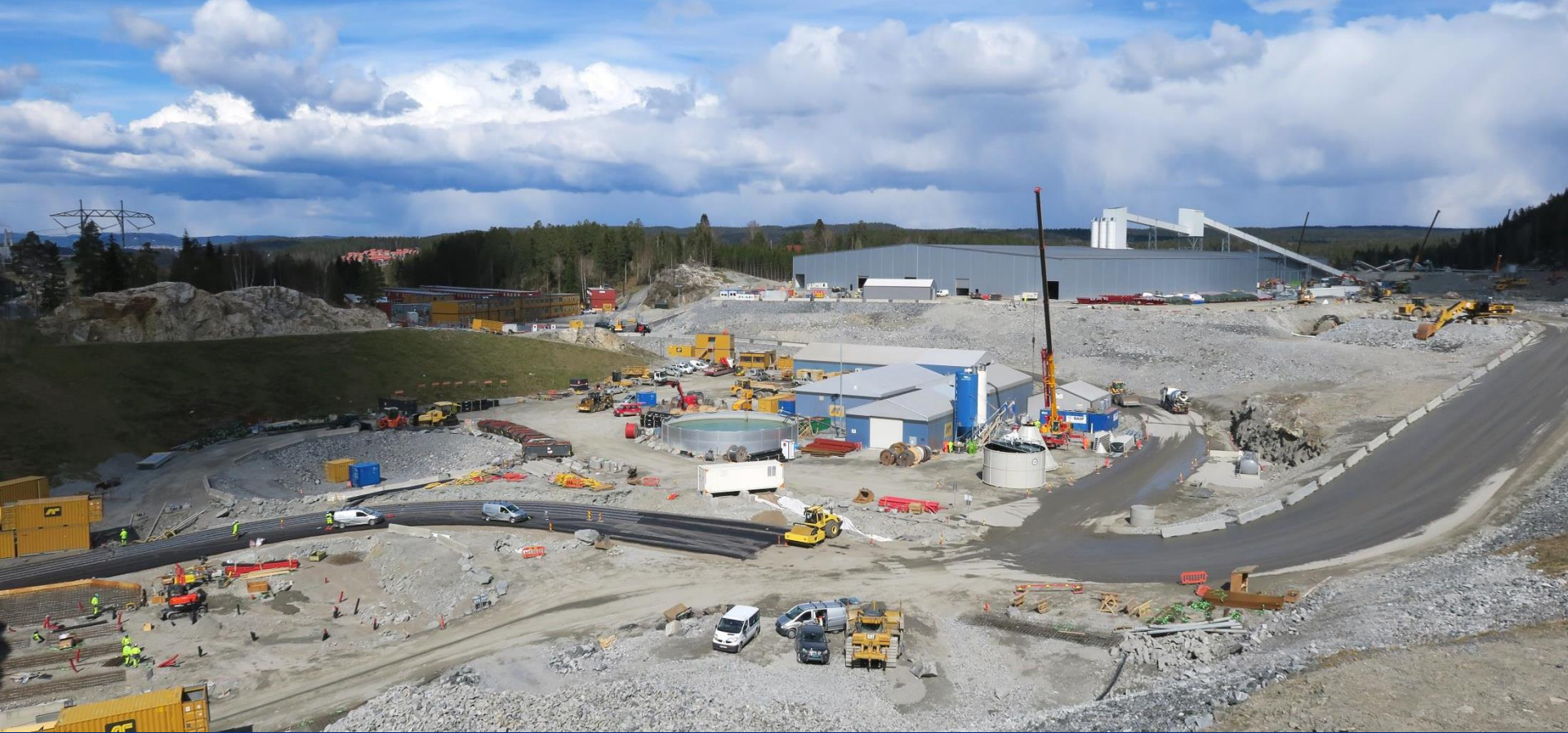
Excavated material will be reused at Åsland rig area and for segment production
