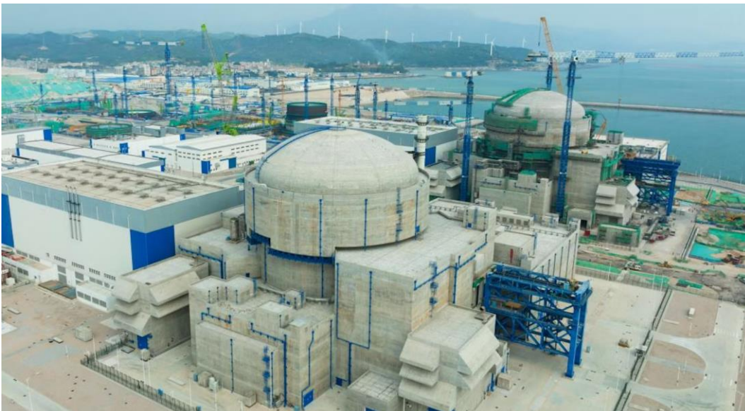
Figure 2.9: Zhangzhou-1 is the first of four Generation III Hualong One units planned for the site in eastern China (CNNC, 2025)
