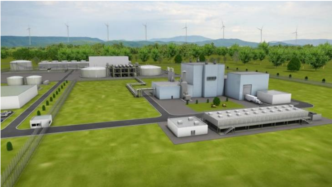
Figure 2.26: Rendering of the Site Arrangement for Deployment of the Sodium Reactor (TerraPower, 2025)
