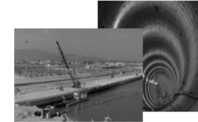
Marine and tunnelling works
