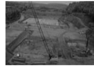
Earthworks, site preparation and temporary infrastructure
