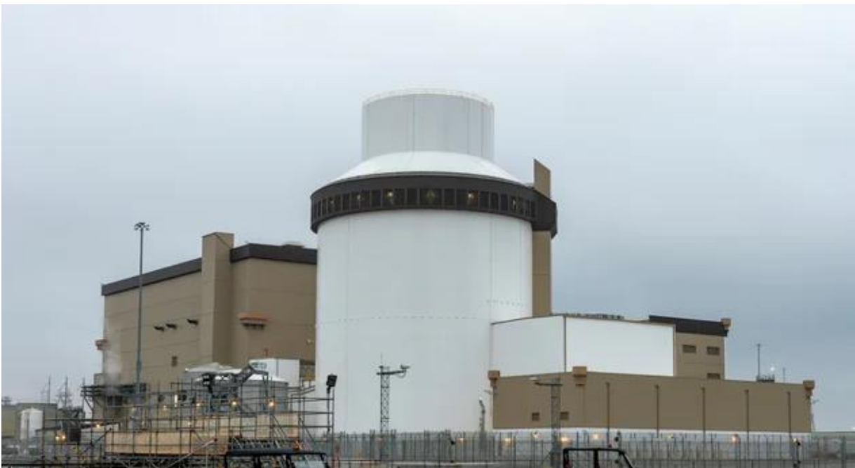
Figure 2.3: AP1000, Unit 3 at Vogtle, US (Westinghouse, 2023)
