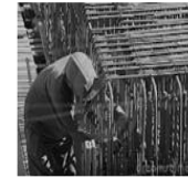
Civil construction and construction support
