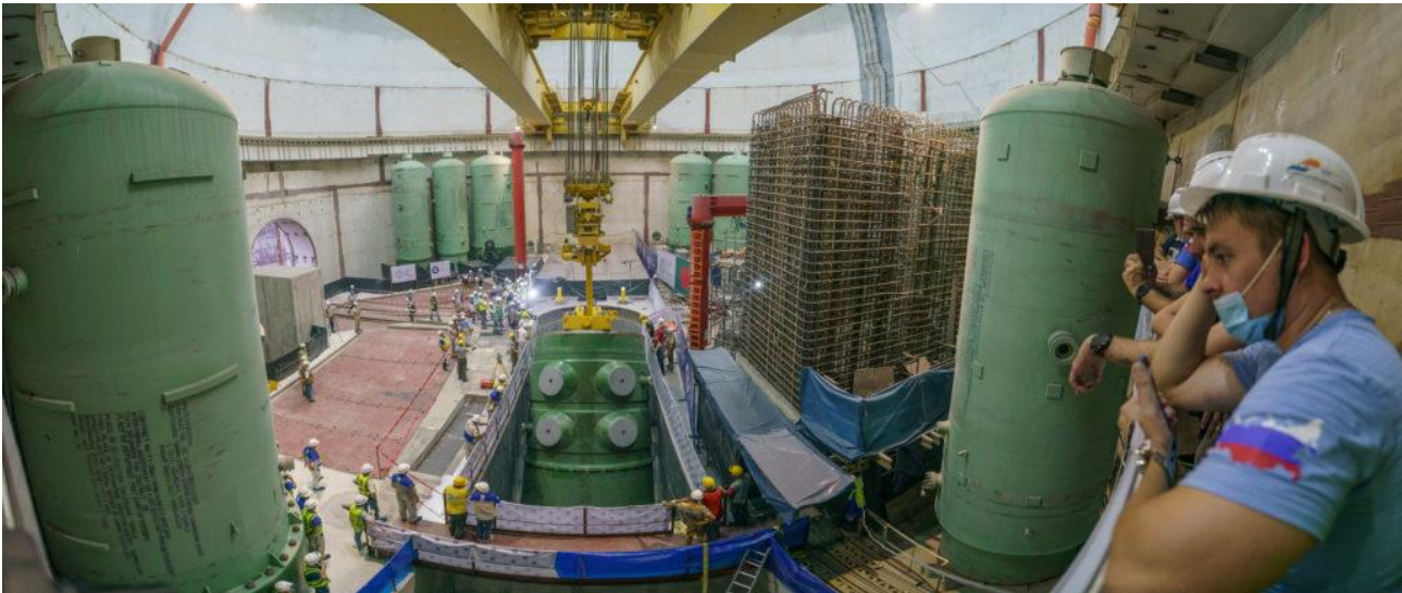
Figure 2.10: Inside a VVER-1200 Reactor Building During Construction (Atommedia, 2025)
