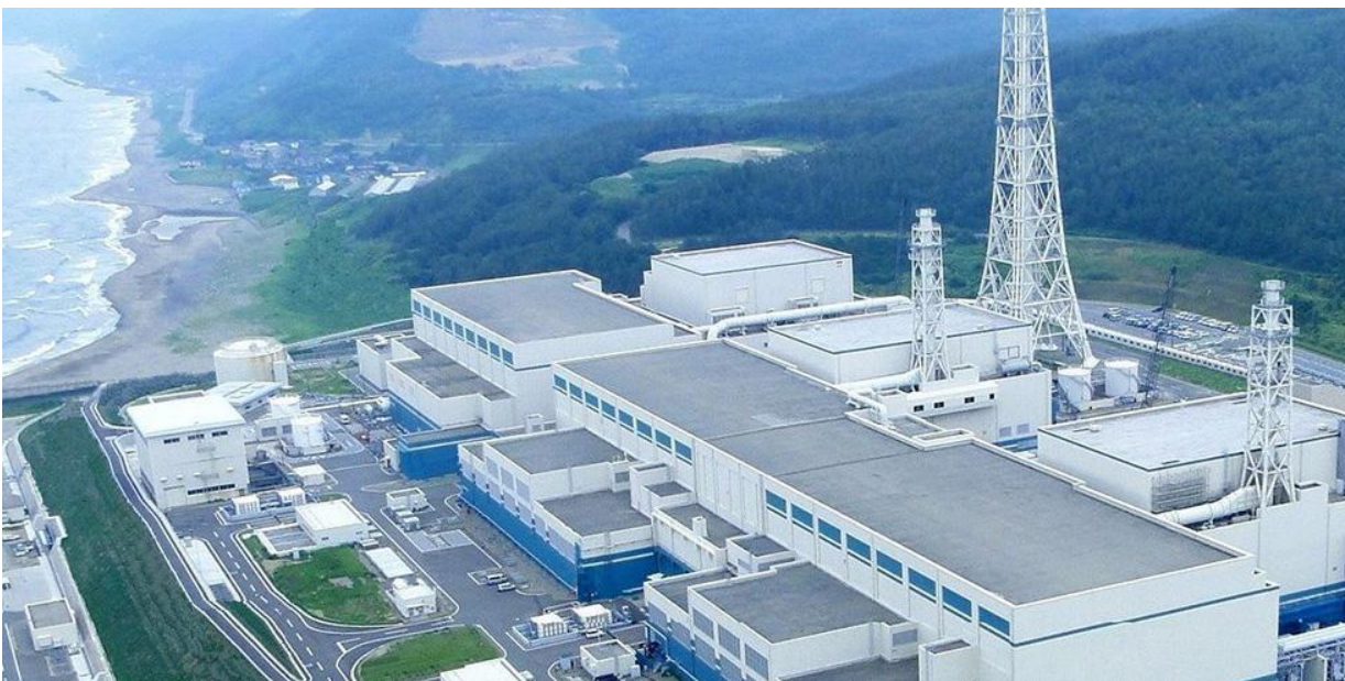
Figure 2.5: Units 5 BWR and 6+7 ABWR of the Kashiwazaki-Kariwa plant (TEPCO, 2025)
