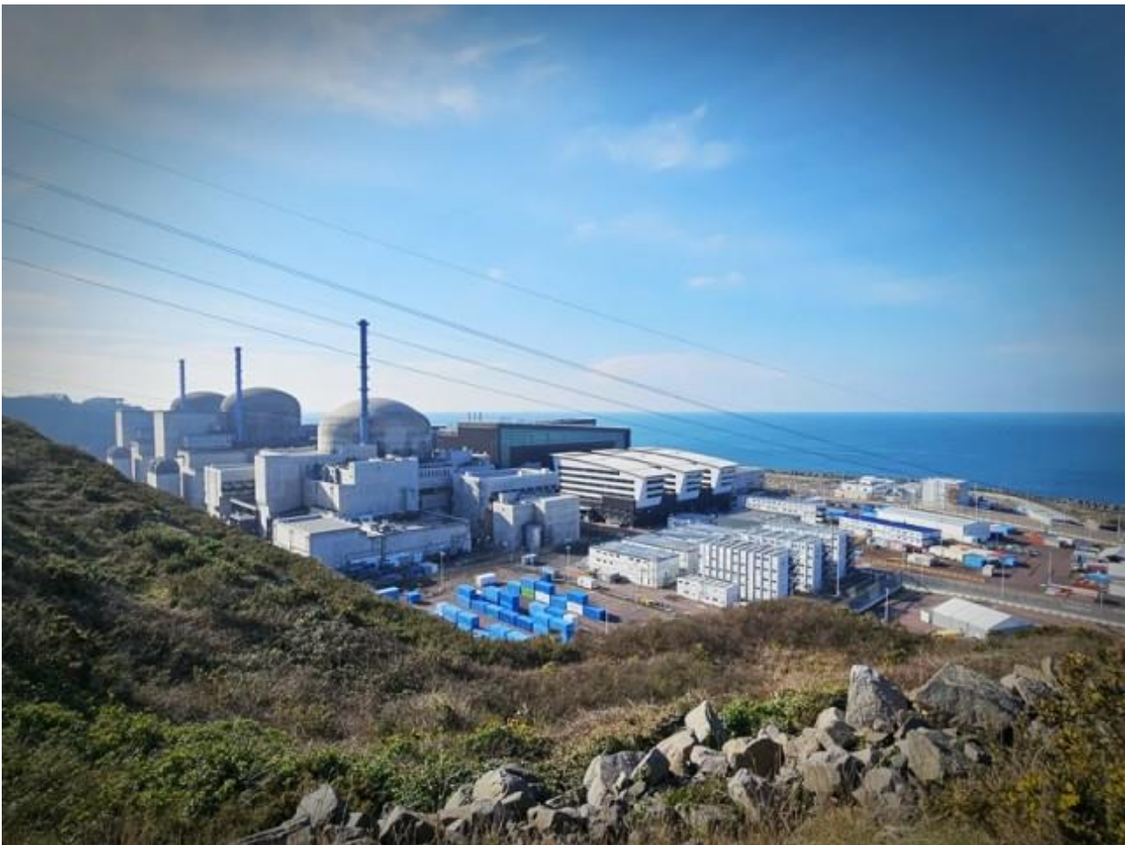
Figure 2.6: EPR in foreground of 2 older units at Flamanville, France (EDF, 2025a)
