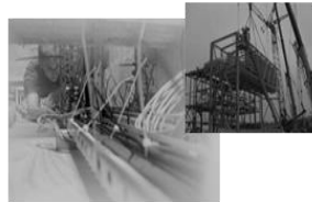
Mechanical and electrical erection
