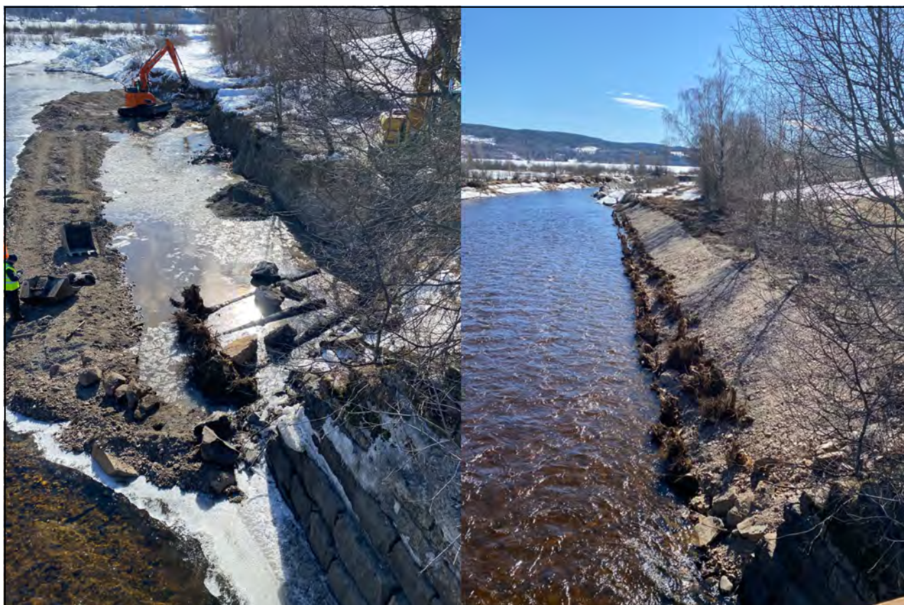
Figure 4.2 Nature-based solutions – stabilisation of stream banks to prevent erosion
