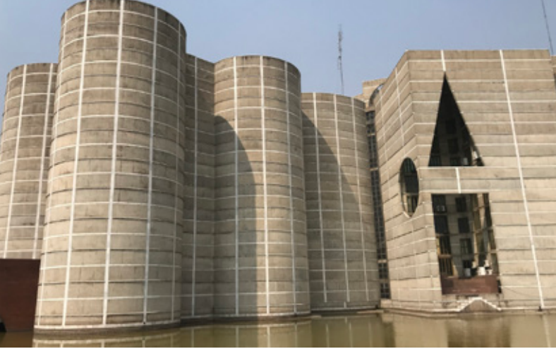
The Parliament building in Dhaka (Photo: Kristin T. Wæringsaasen)
