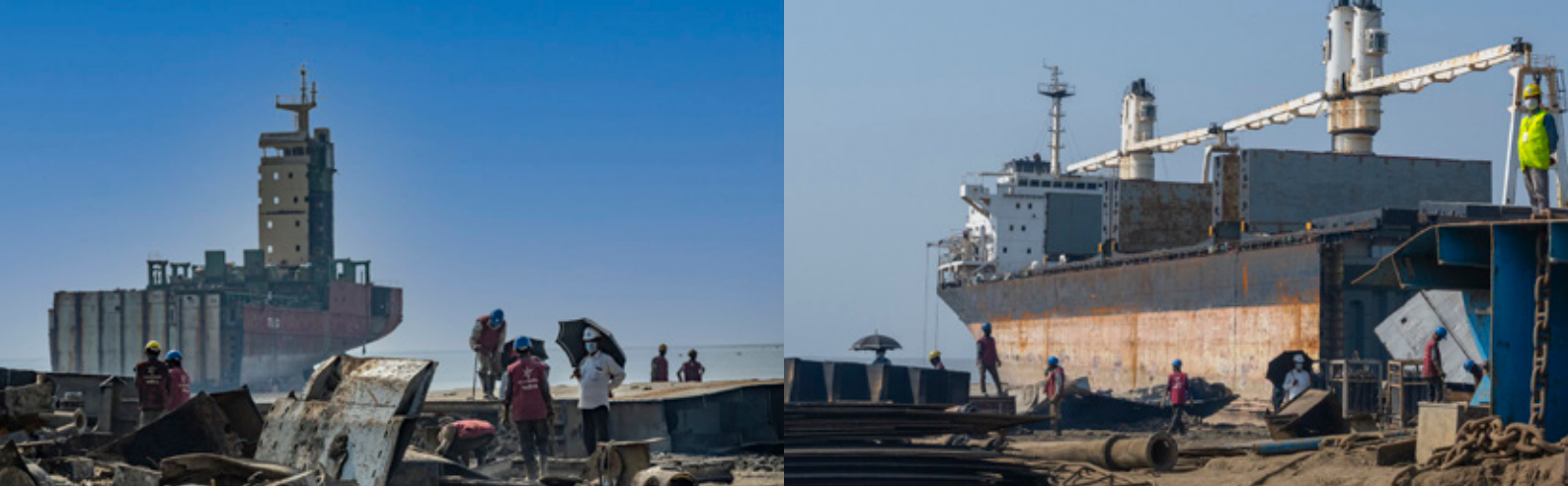
Ship-breaking and recycling is an important income-earning business, taking place on the shores near Chattogram. Norway supports a project by the International Maritime Organization (IMO) to make this activity safe, environmentally sound and sustainable in line with international standards. (Photo: E. Rikter-Svendesen)
