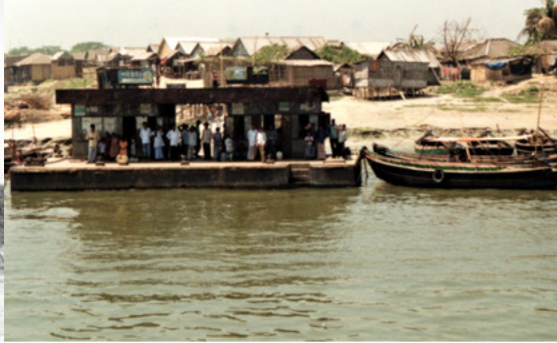
Pontoons, floating jetties, were essential for access to the river boats. They were flexible and adjusted to fluctuating water levels and when the rivers changed direction. Picture from 1994. (Photo: Arve Ofstad)
