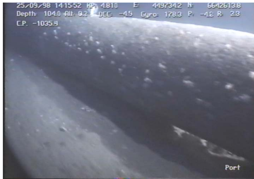
Figure 2.3 Free span on pipeline
