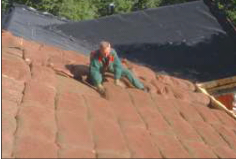
Lay the mesh bags close together.
