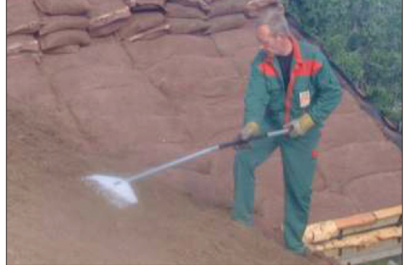
At the end the roof is leveled with peat before watering.
