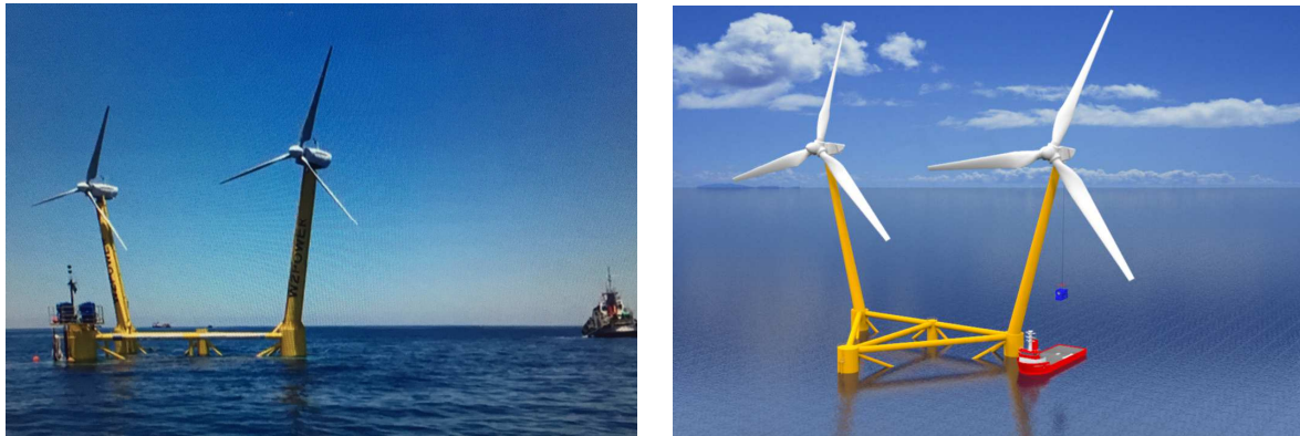
Fig. 4. (Left): W2Power prototype installed at sea off Gran Canaria 17.06.2019, notice tug boat leaving in background. (Right): render of the full sized 12MW W2Power. Servicing vessel and large piece being lowered onto it shows scale.
